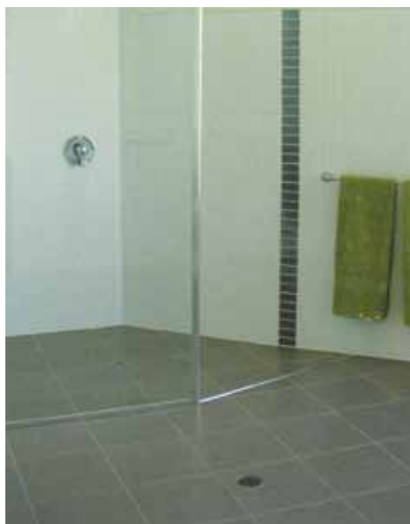
An example of a shower with a level entry
