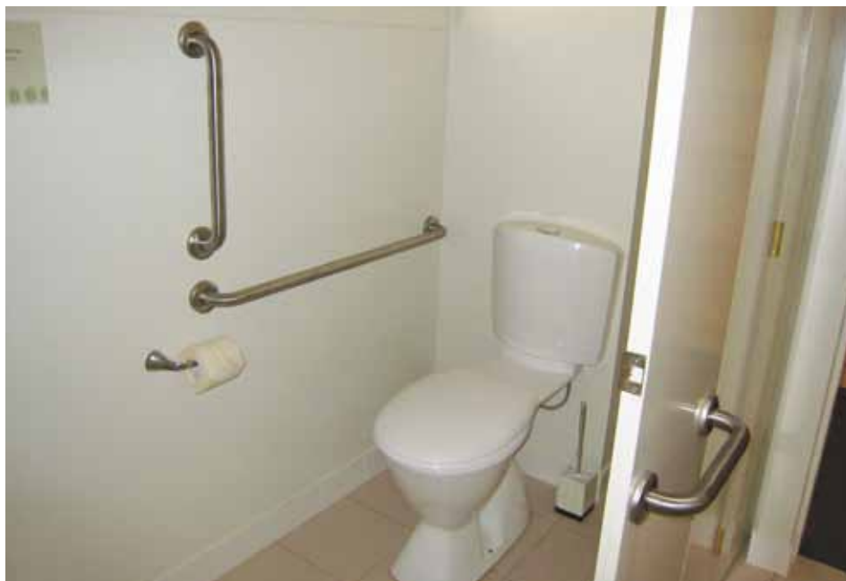
Grab rails attached to the wall provide leverage and stability
