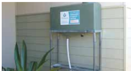
An example of a greywater treatment system
