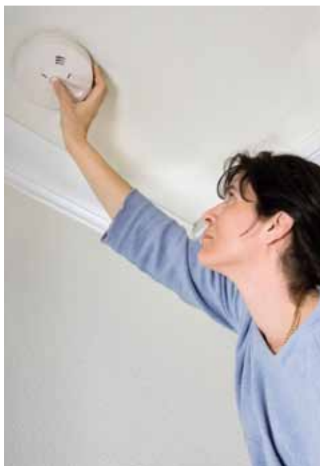
If your home was built before 1 July 1997 it will require at least one 9-volt battery powered smoke alarm
