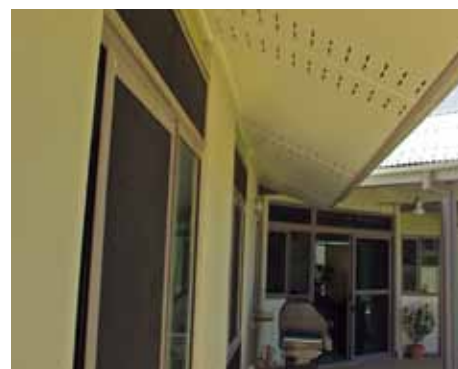
Wide eaves that have vents can reduce heat from the sun by shading windows and help ventilate your home
