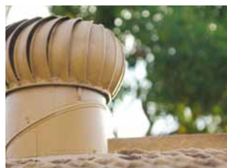
Whirlybirds are a good example of roof ventilation
